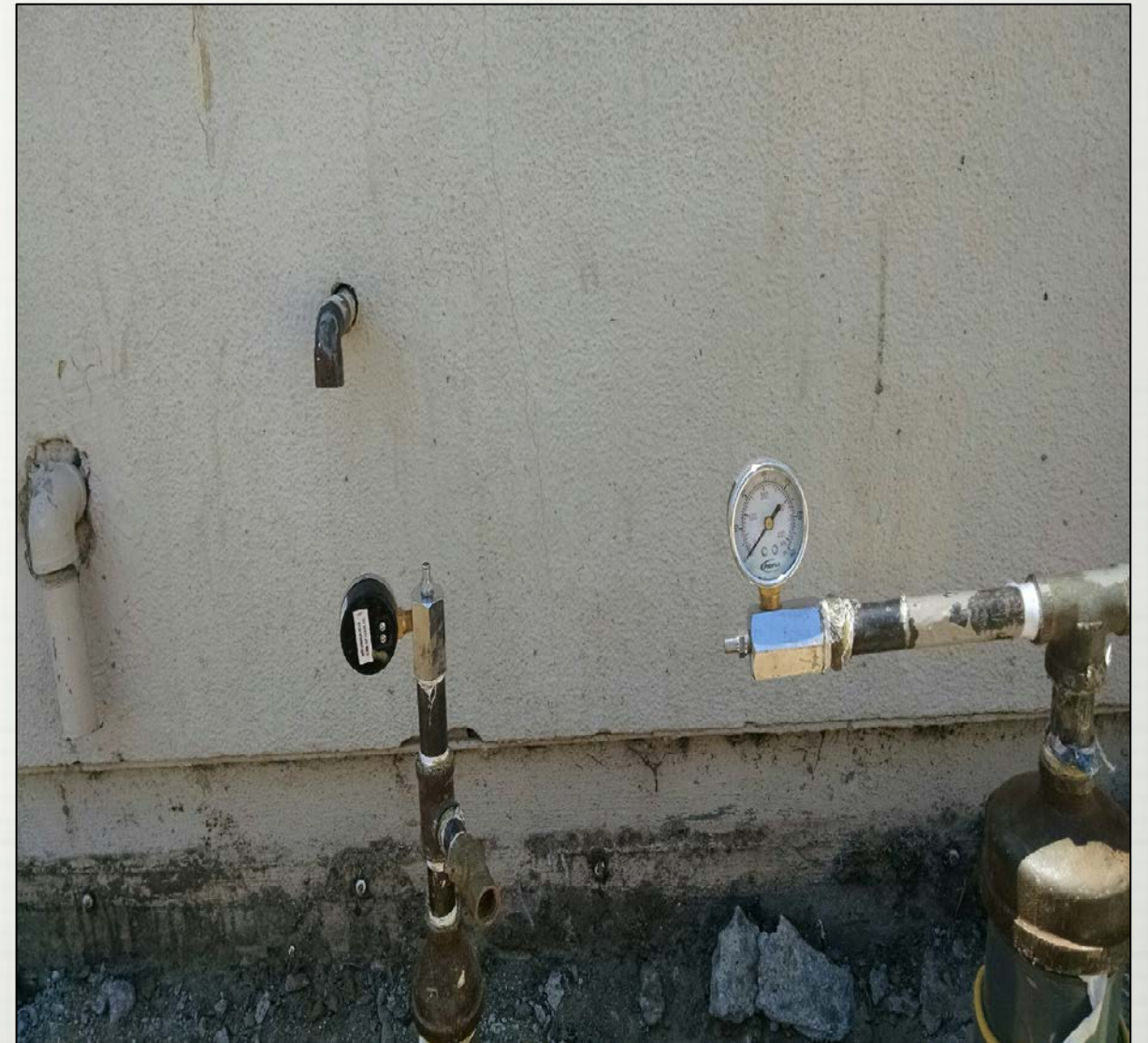
Storm drain tie in and gas line pressure testing
